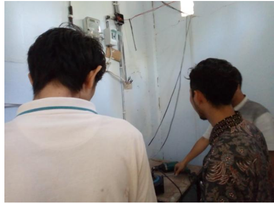
Gambar 4. Proses instalasi inverter
