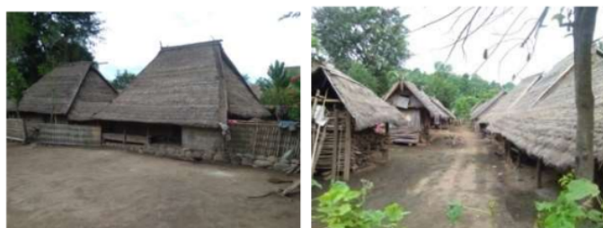
Figure 10. Traditional houses in Dusun Beleq: walls were made of Gigantochloa apus , roofs made of Imperata cylindrica , and pillars made of Gigantochloa atter , Toona sureni , Artocarpus heterophyllus or Swietenia macrophylla
