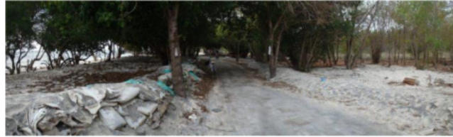
Fig. 5. The condition in south and west side.
