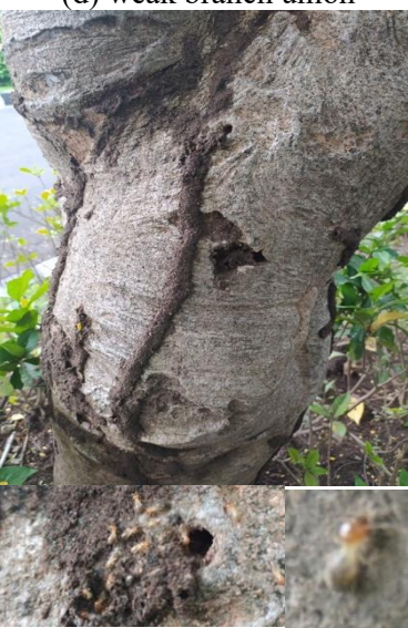
(g) termite attack
