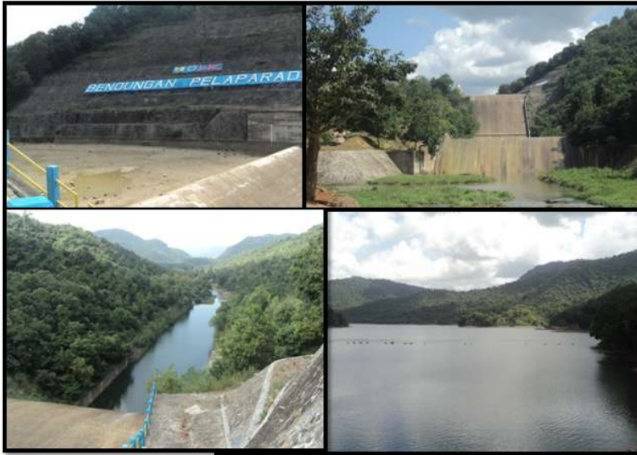
Figure 2.1 Condition of Pelaparado DAM in Pelaparado Watershed Of Sumbawa River Basin
