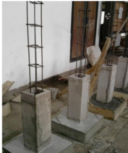
Figure 4. Column specimen preparation.
