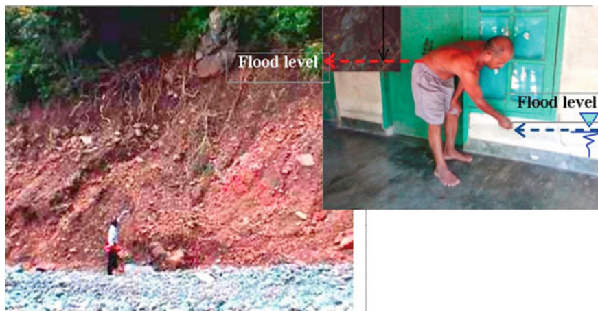
Fig. 3 Flood level-marking based on personal information (Courtesy of West Lombok public works and housing office, 2017)
