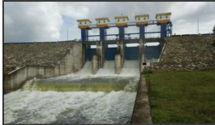
Fig. 1. The Pandan Duri dam located in the East Lombok District of the West Nusa Tenggara Province, Indonesia.
