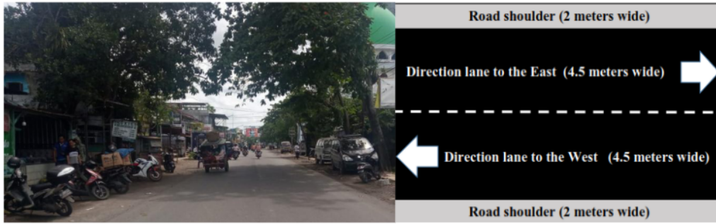
Figure 1. Condition of section road without median type 2/2 UD
