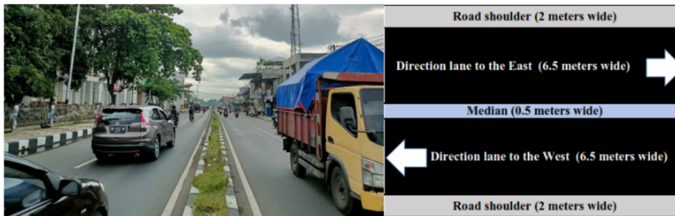
Figure 2. Section road condition with median type 4/2 D
