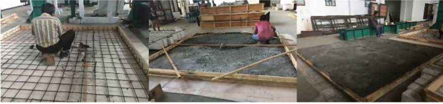
Fig. 2. (a) Strain gauge installation, (b) casting, and (c) slab specimen.
