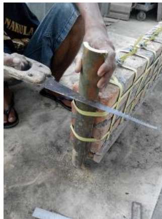
Figure 3. Slipping the bamboo under the PP-band mesh
