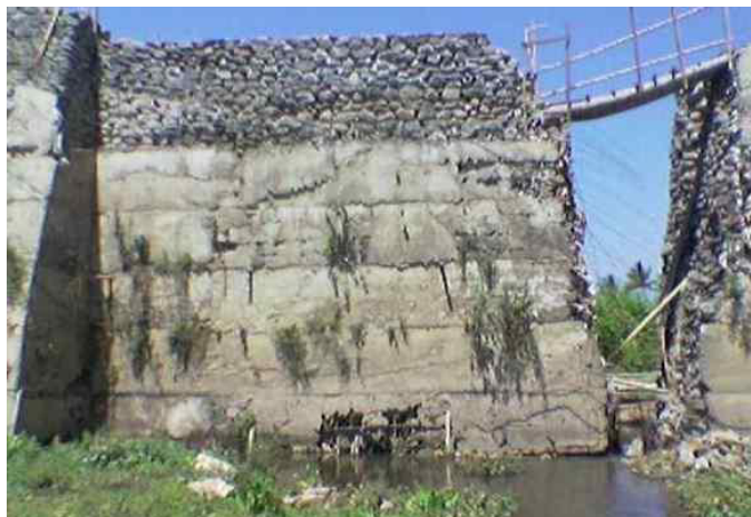
Figure 15. Additional height with different materials (Courtesy of BWS NT I)
