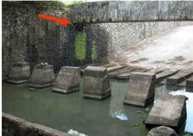
Figure 11. Leakage at the vertical wing wall of stilling basin (Courtesy of BWS NT I)
