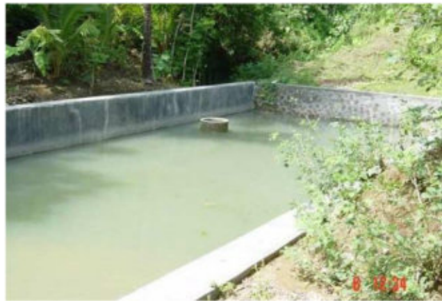
Figure 2. An embung desa with masonry structure as its embankment (Courtesy of BISDA NTB)
