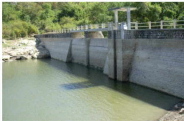
Figure 3. An embung pemerintah equipped with adequate intake and spillway (Courtesy of BWS NT I)
