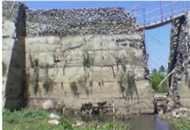
Figure 15. Additional height with different materials (Courtesy of BWS NT I)
