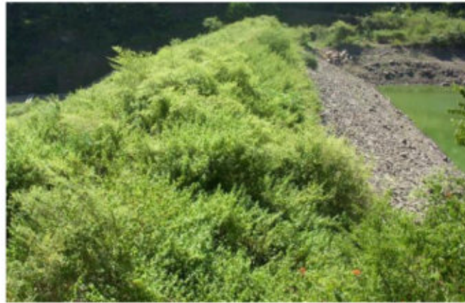
Figure 5. Undesirable vegetations cover the top and downstream slope of embung (Courtesy of BWS NT I)
