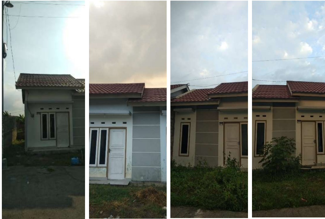
Gambar 4. 7 Lokasi pemasangan blok B.26, C.19, D.17, D.16
